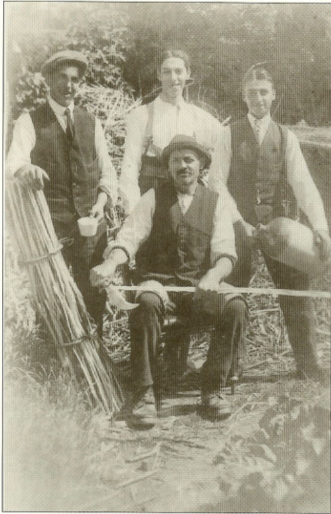
Plate 35 – George Tuck, the village thatcher, seated in front of his son Fred Tuck (right) and Frederick Watts (left). To the left is a bundle of the lathes or spars that he made for keying in thatch on roofs or ricks.
